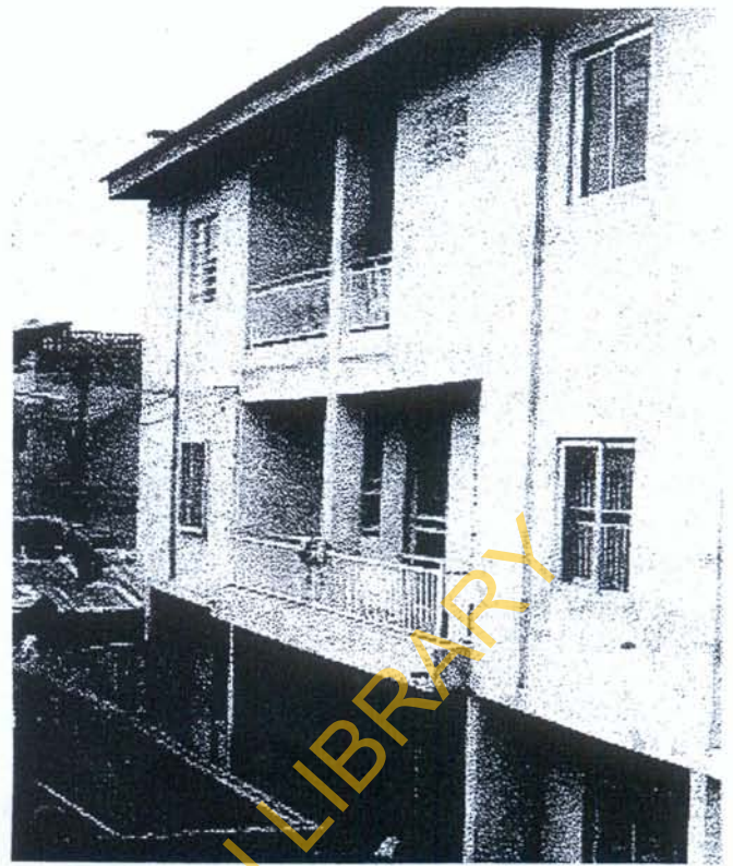
Figure 8. A six-flat apartment building in Yemetu, Ibadan Source: Field survey, June 1997
