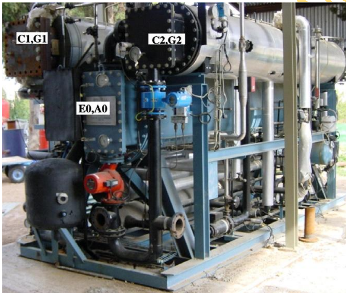
Fig. 2d. Typical two-stage Absorption Chiller
