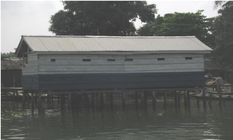
Plate 4.21: Toilet built directly on water body in Sangana community
