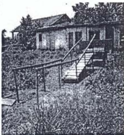
Plate-2 : the completed ramp.
