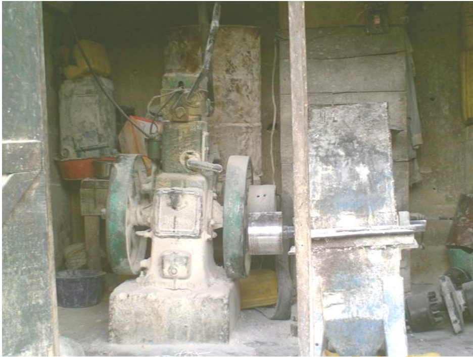
Plate 11: Milling machine in Bódijà Market. (Source: Fieldwork 2010)
