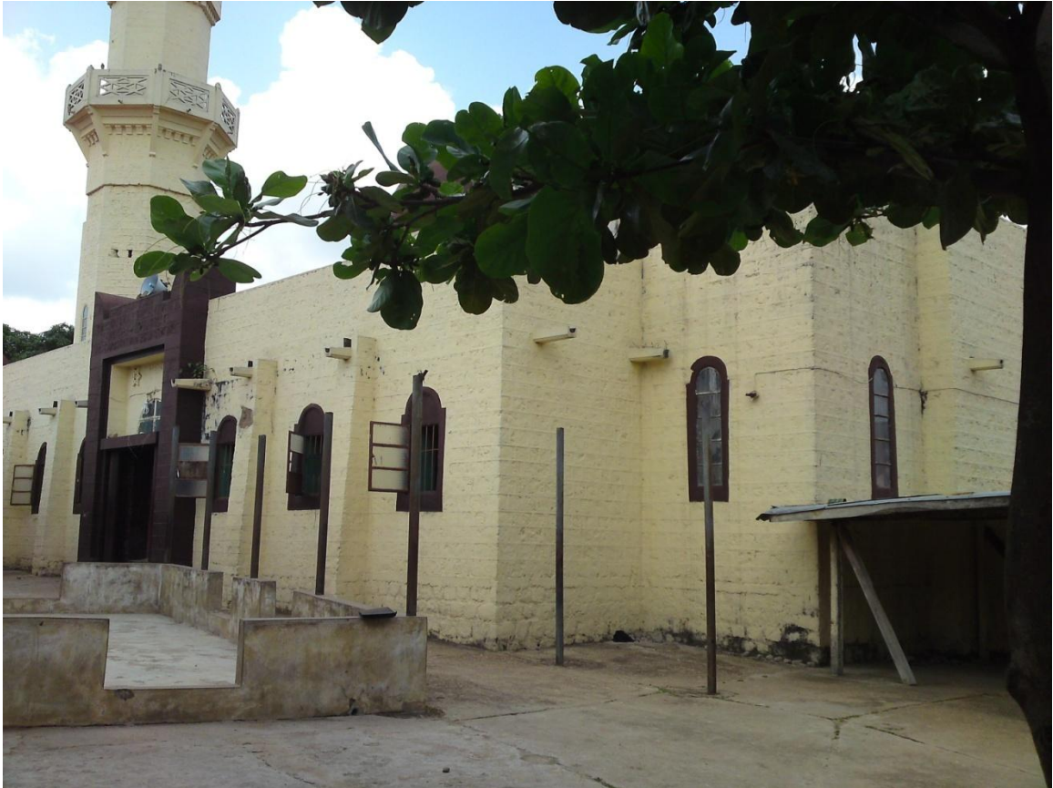
Picture 9: Okene Central Mosque (The First Central Mosque in Ebiraland )
