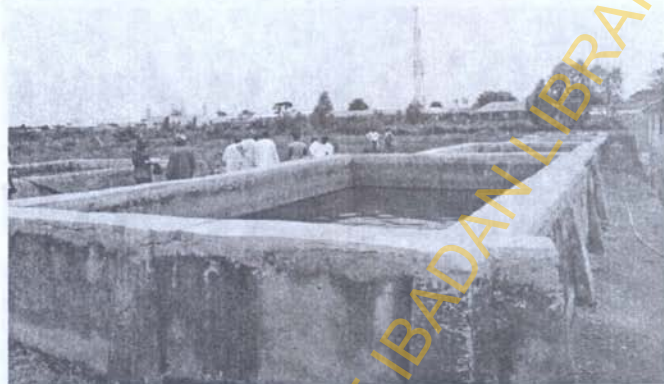
Fig. 7: Concrete tanks used as extensive fish culture system
