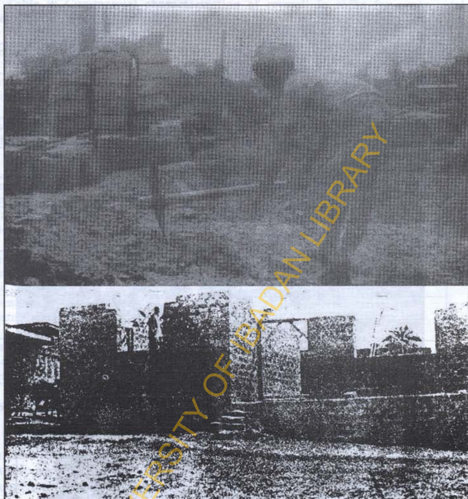
Fig. 11: Exploitation of lateritic clay for simple sun-dried bricks in building of low-cost accommodation
