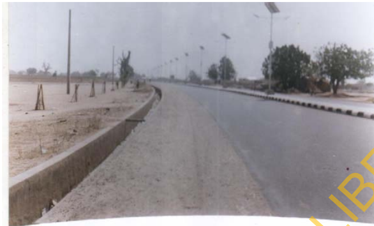
Plate 4: Newly Planted Trees Protected from Vandals and Animals along Potiskum to Gujba Bypass Road, Damaturu
