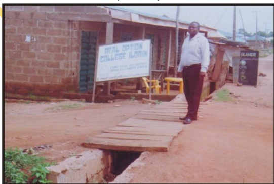
Construction of Culvert and Rehabilitation of Street Odota Community, Ilorin. (Plate 15)
