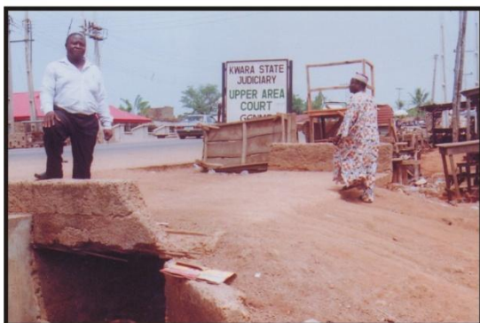
Construction of Culvert at Ganmo Ifelodun L. G. (Plate 9)
