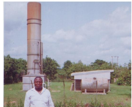
Maintenance of Water Works by Ira Community For sustainability Ifelodun L. G. (Plate 6)
