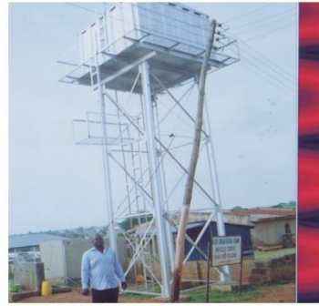
Gaa-Odota Community Bore Hole Ilorin West L. G. (Plate 18)
