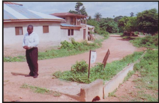
Construction of Drainage and Rehabilitation of Street, Ik A Community (Plate 44)
