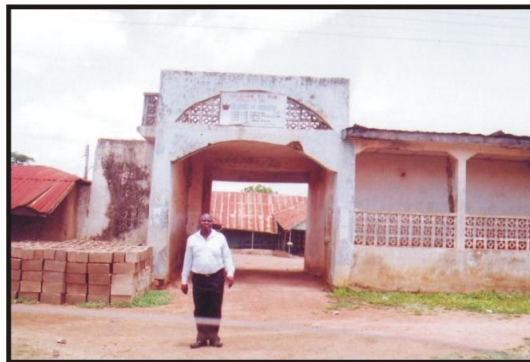
Construction of Omupo Community Palace Ifelodun L. G. (Plate 3)
