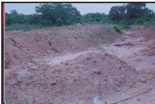
Construction of Drainage Obagun Community (Plate 39)
