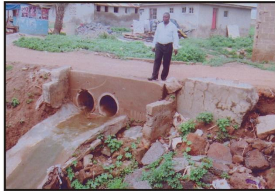
Construction of culvert and Road rehabilitation at Gaa Area, Ejigbo. (Plate 50)
