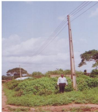
Extention of Electrification Poles at Oke-Itunu Community, Ejigbo Osun State (Plate 37)
