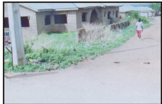
Rehabilitation of Road at Seke Community, Ifelodun L. G. (Plate 48)
