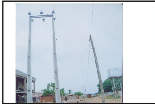
Akinlabi Community Extention of Electrification Poles (Plate 45)
