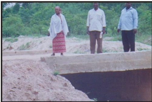
Bridge Construction at Lanwa Community Moro L. G. (Plate 29)
