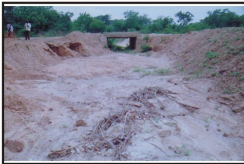
Construction of Drainage at Onikoko Moro L. G. Kwara State. (Plate 31)
