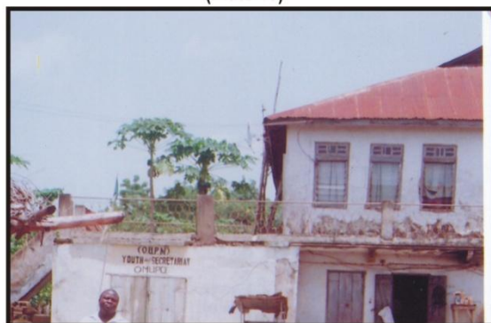
Omupo Community Cooperative Building Ifelodun L. G. (Plate 12)
