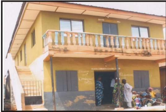
Laase Community: Erection of Building for Community Based Organisation Centre (Plate 43)
