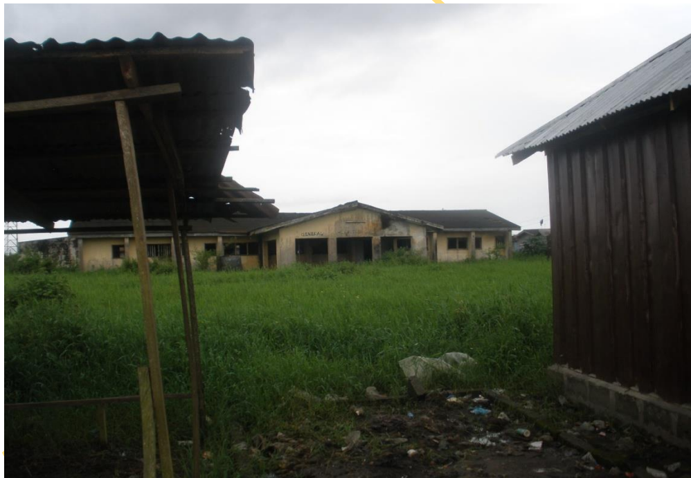
Plate 5: 3 Abandoned general hospitals in Igbokoda (Ilaje LGA)
