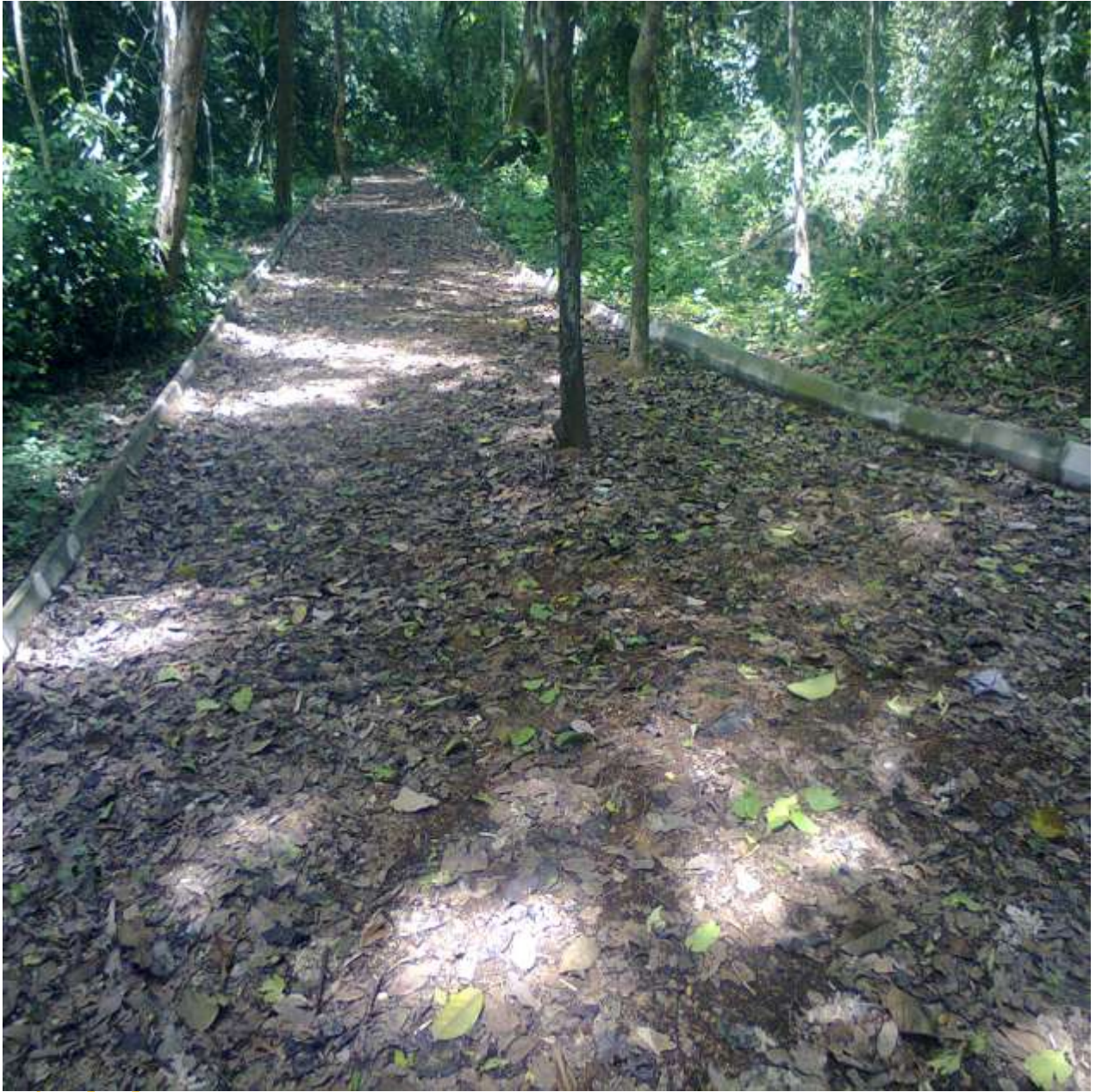
Plate 16: The Newly Constructed Walk Way inside OOWHS.
