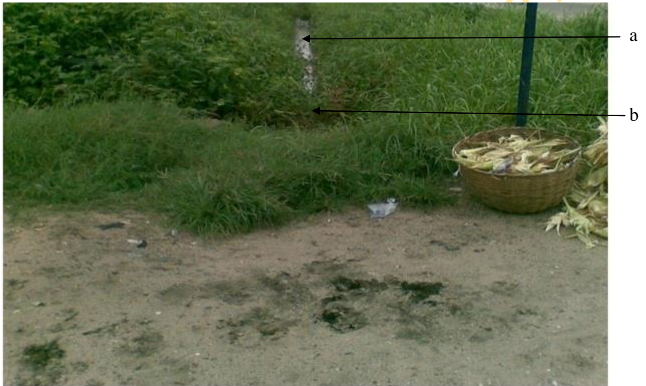
An occluding wastewater drain on Ahmadu Bello Road in June, 2004 with (a) gradual loss of habitat to wastewater fauna including P. reticulata and (b) fully blocked section.
