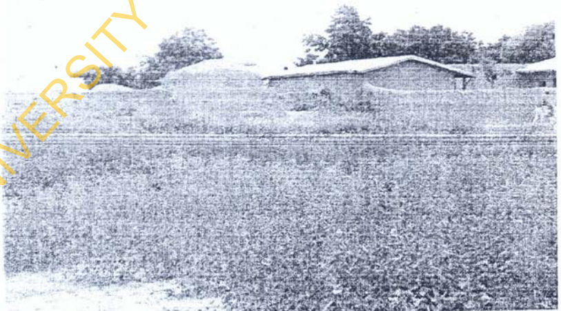
Fig. 22: Mud houses in Birni Tsaba Community in Zurmi LGA of Zamfara State. Note the mixture of round mud roof and double-pitch roof made of corrugated metal sheets.
