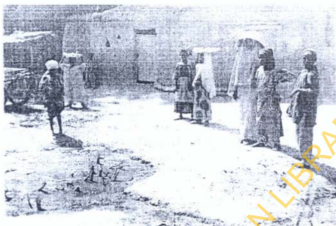
Fig. 28: A rural mud house in Modomawa Community in Birni Mogaji LGA of Zamfara State. Note the entrance door made of corrugated zinc roofing sheet, and the two rectangular openings to monitor the outside from inside the house. In the foreground is a pit containing waste water from a UNICEF-assisted hand-pump well. Sugar-cane is planted in the pit to utilize the waste water. (Source: Author, 12/9/07)
