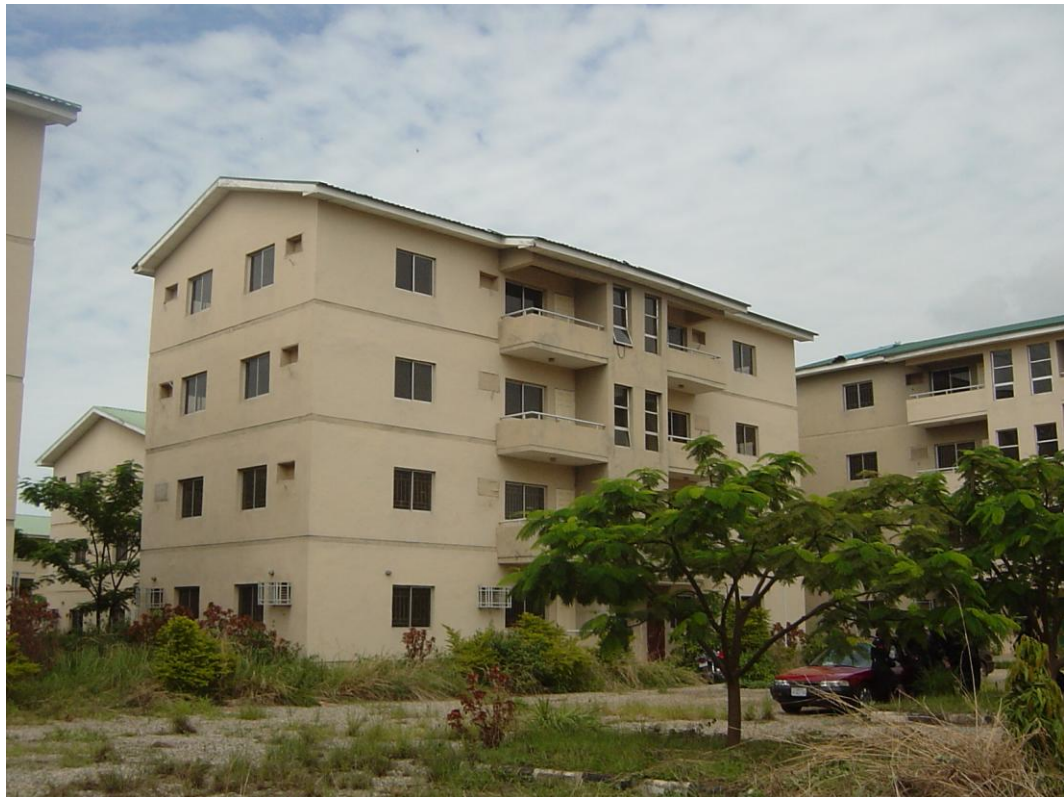
Plate 28: Newly built barracks for Police in Abuja and some states in the country under the Federal Mortgage Bank/Police Loan Scheme.
