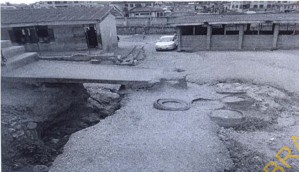
Plate 3: Gully Erosion at Eleta High School, Ibadan Southeast Local Government Source: Authors' Survey, 2014
