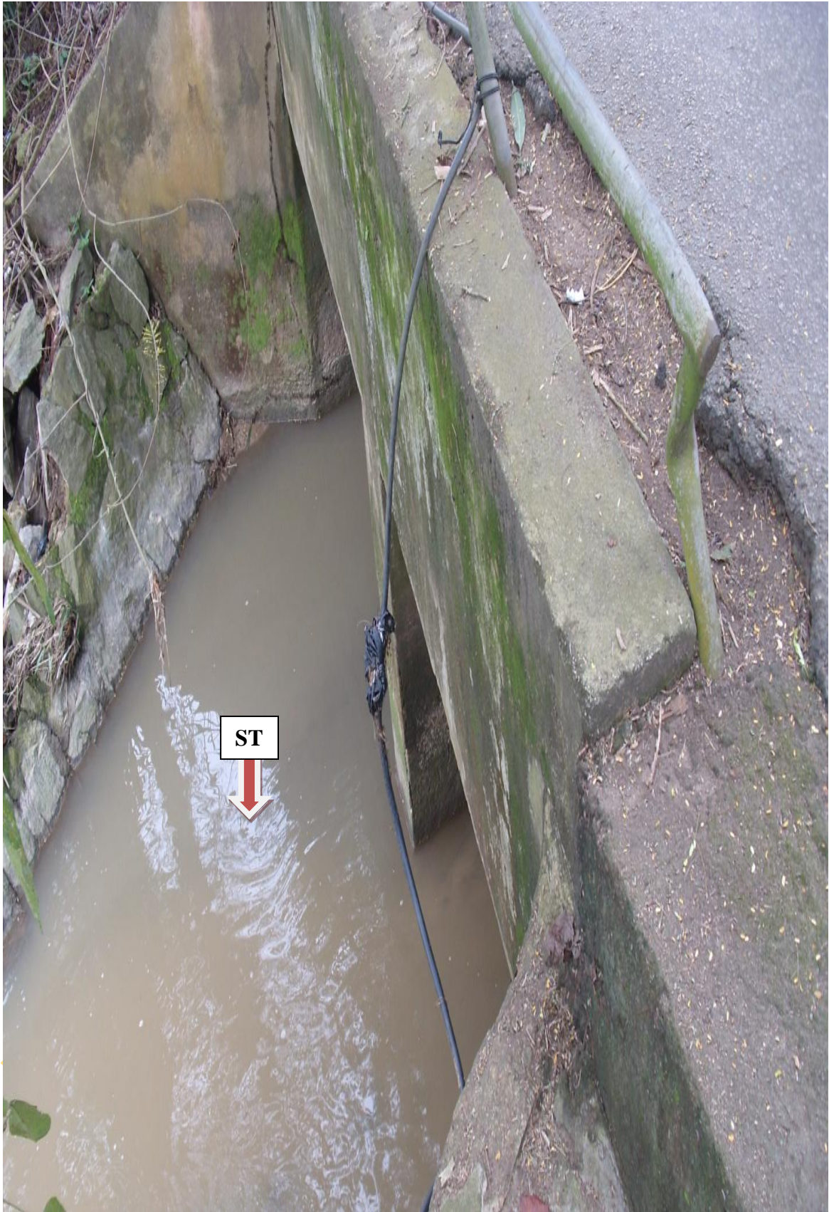
Plate 3.11: Control stream (Awba stream, UI)
