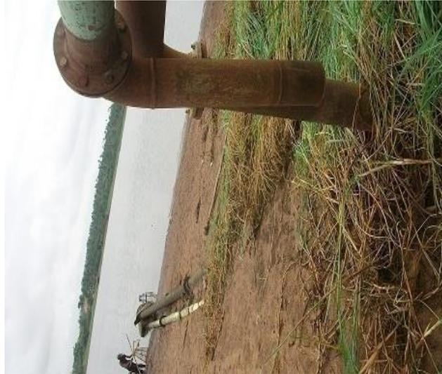
Exposed underground pipes at Oyo and Osun axis of Asejire dam catchment after Lakes' water was drawn-down
