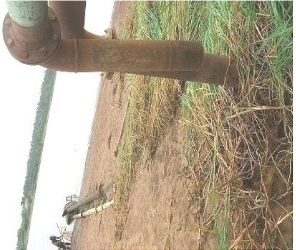
**Plate 10b: Rusting underground pipe of water pumping station on O<sub>s</sub>S strata of Asejire Lake (Exposed when water level was drawn down- October, 2010)**
