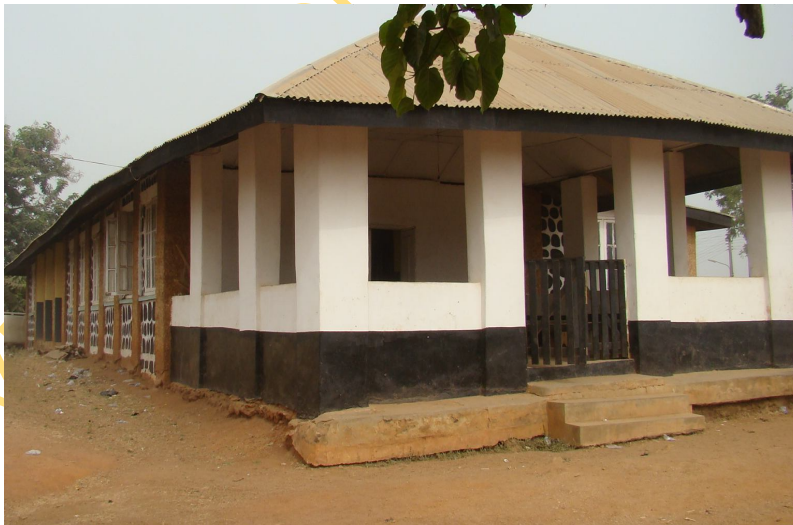
Figure 13.13 Local Government Maternity Centre in Oke-Ola Oro Town
