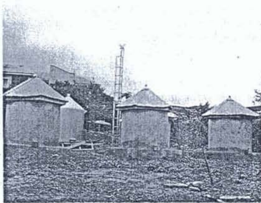
Plate 1a. A group of termite mound clay silos
