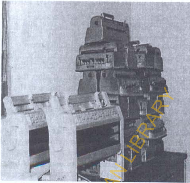
Fig. 7: Braille embosser and Perkins Brailler
