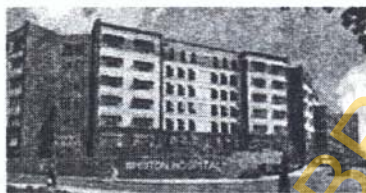
Mersey Regional Burns and Plastic Surgery centre at Whiston Hospital
