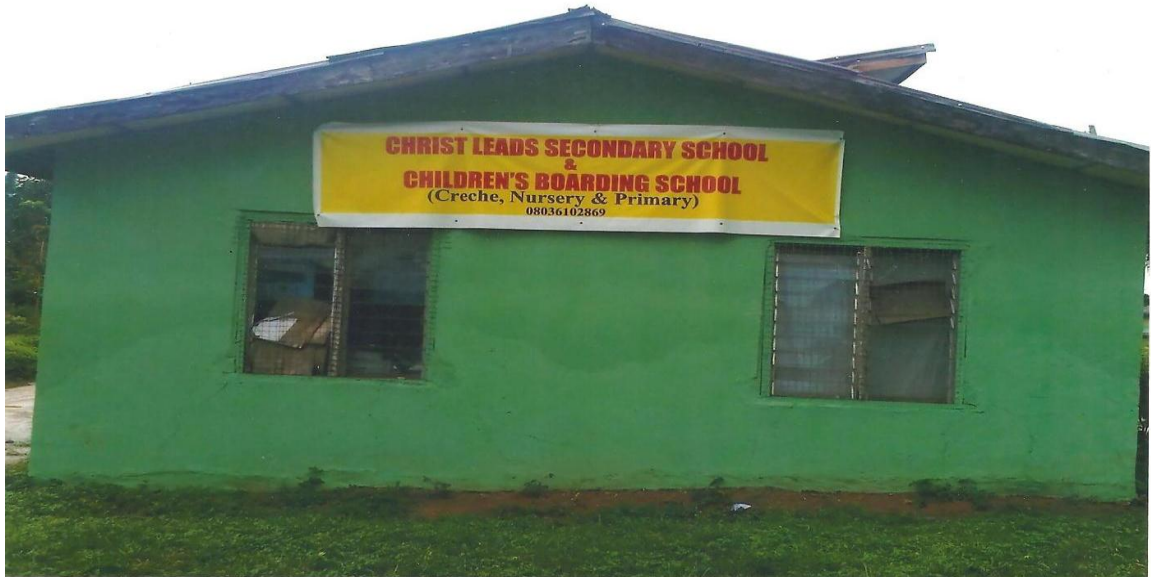
Administrative Block at Children Boarding School, City of Life Camp, Fadeyi Estate, Osogbo.
