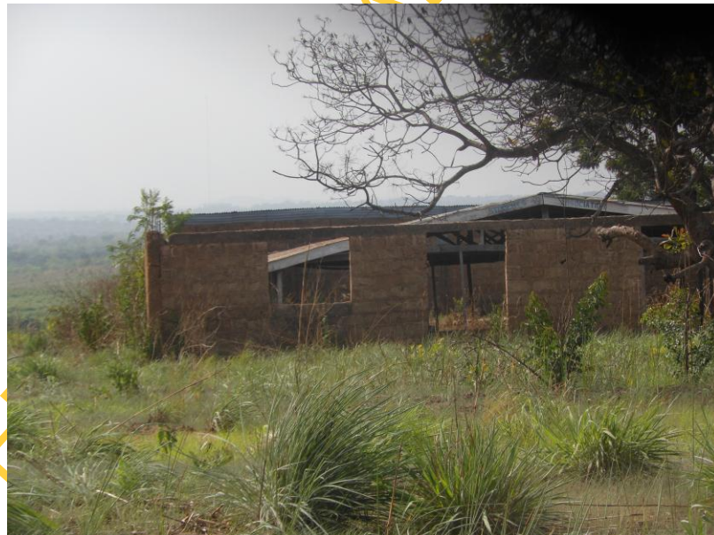
The Structure used by Christ Apostolic Church Students' Association (CACSA)
