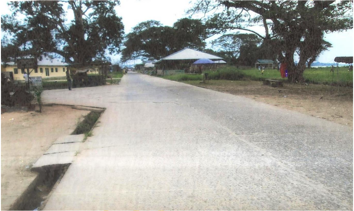
Plate 12. Internal Concrete Link Road, Odi
