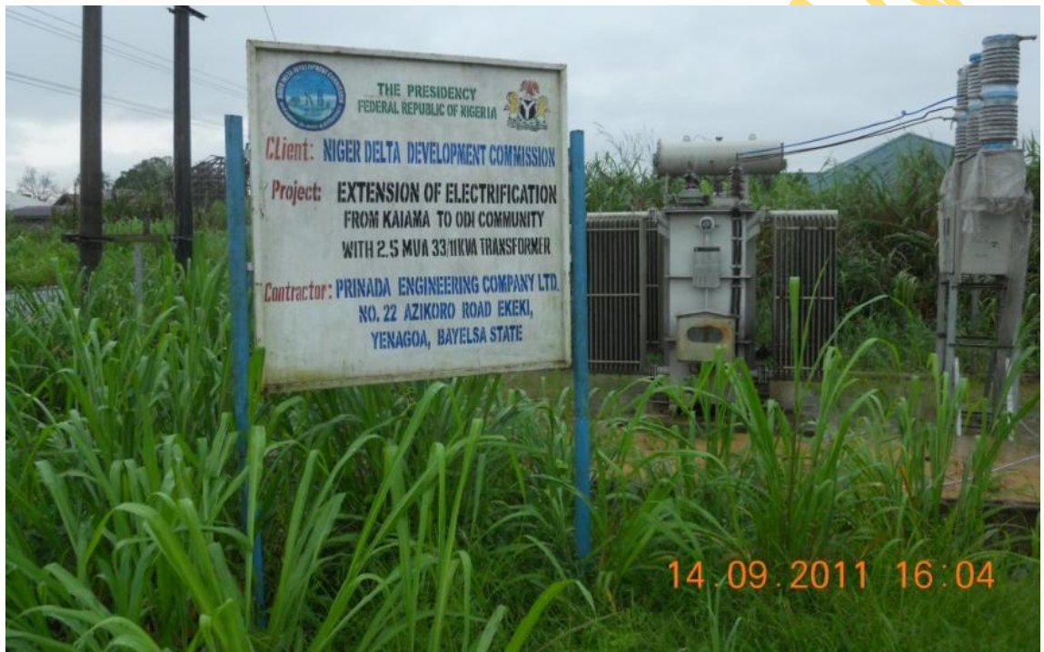
Plate 8. Rural Electrification Project
