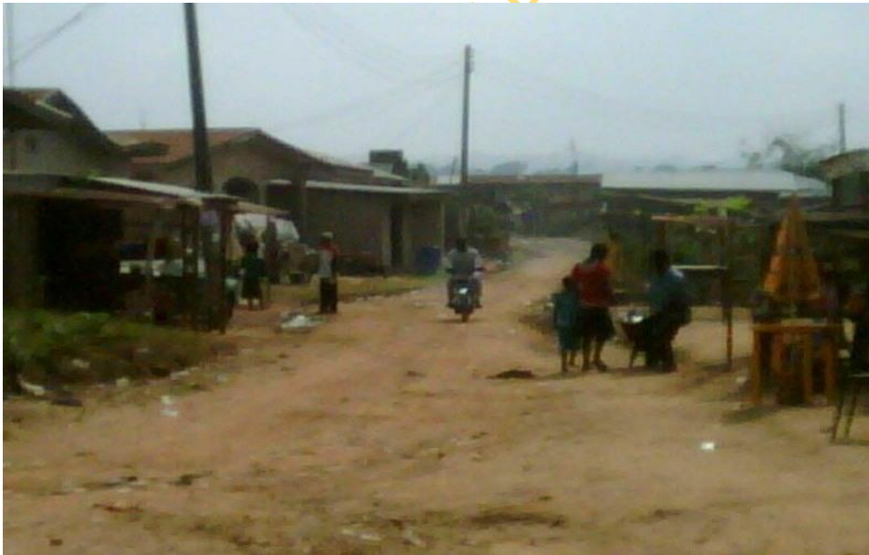
Plate 4: Scene of a Street layout in Apata, with blocks of bungalows having 'face-me-I-face you' rooms. A typical example of a neighbourhood where most low-income earners reside within the city of Ibadan (Source: Cecilia Owolabani: Fieldwork, 2012)
