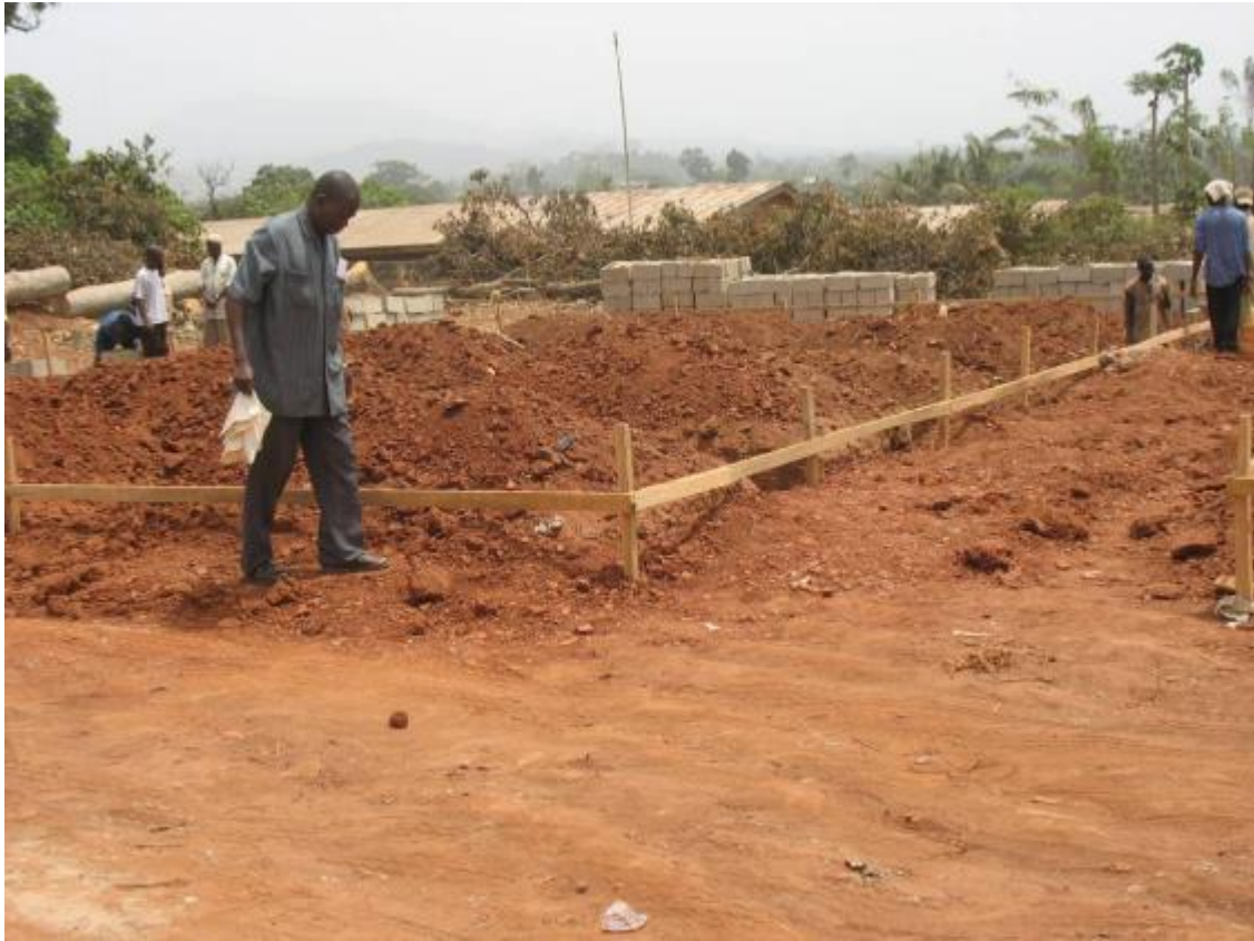
Plate 5.25: A building under construction at Ita-Yemoo, Ile-Ife
