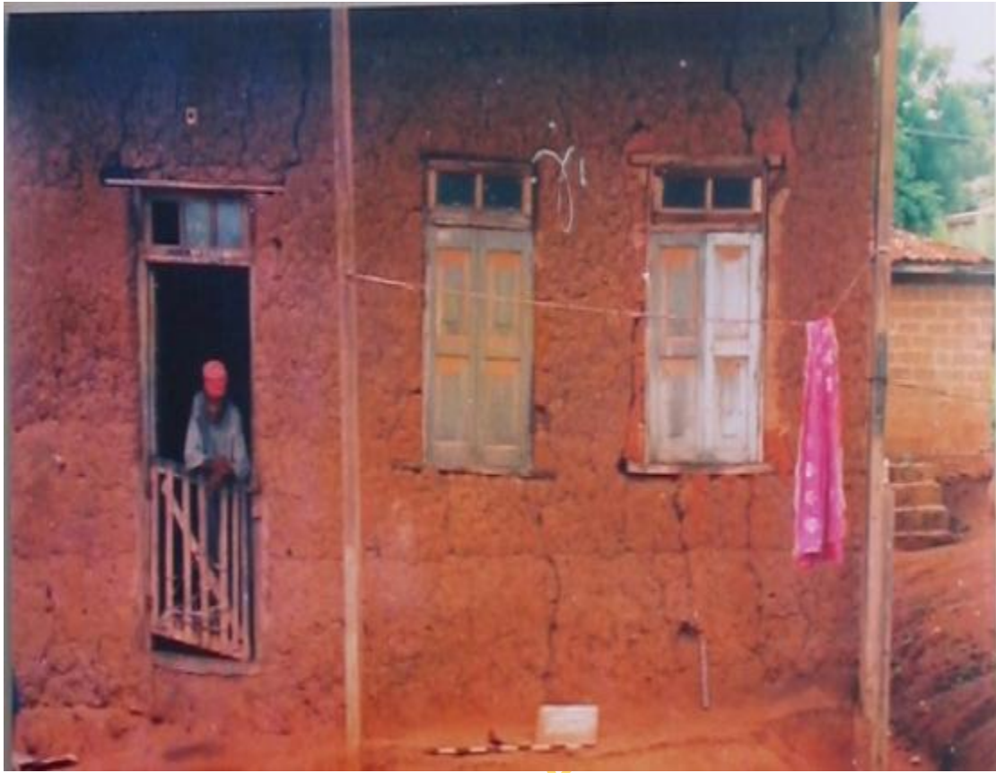
Plate 3.12: A building over the Iragbiji pavement
