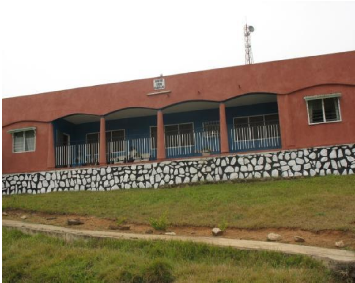
Plate 3.4: Igbajo New palace building
