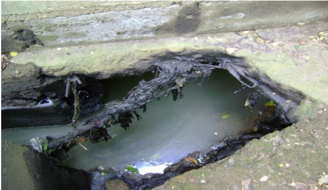
Appendix 2: Effluent channel of Hoesch Pipe Mill Ltd in Ikeja Industrial Estate
