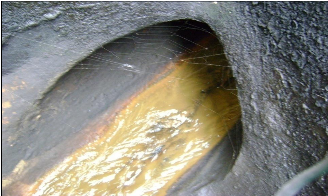
Appendix 4: Effluent channel at the central treatment plant receiving all effluents in Ikeja Industrial Estate.
