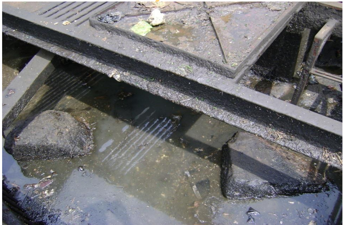
Appendix 7: Effluent channel of PZ in Ilupeju Industrial Estate
