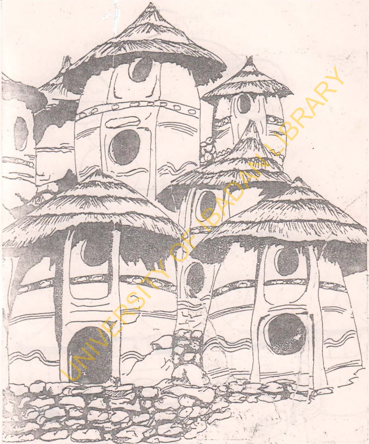
FIG. 62. FOLK-ARCHITECTURE—ROW HOUSE (NORTHERN NIGERIA) MUD WALLS STRENGTHENED WITH LAYERS OF LARGE STONES; DOOR WAY PILLARS AND THRESHOLD REINFORCED WITH STONES, THATCHED ROOFS.
