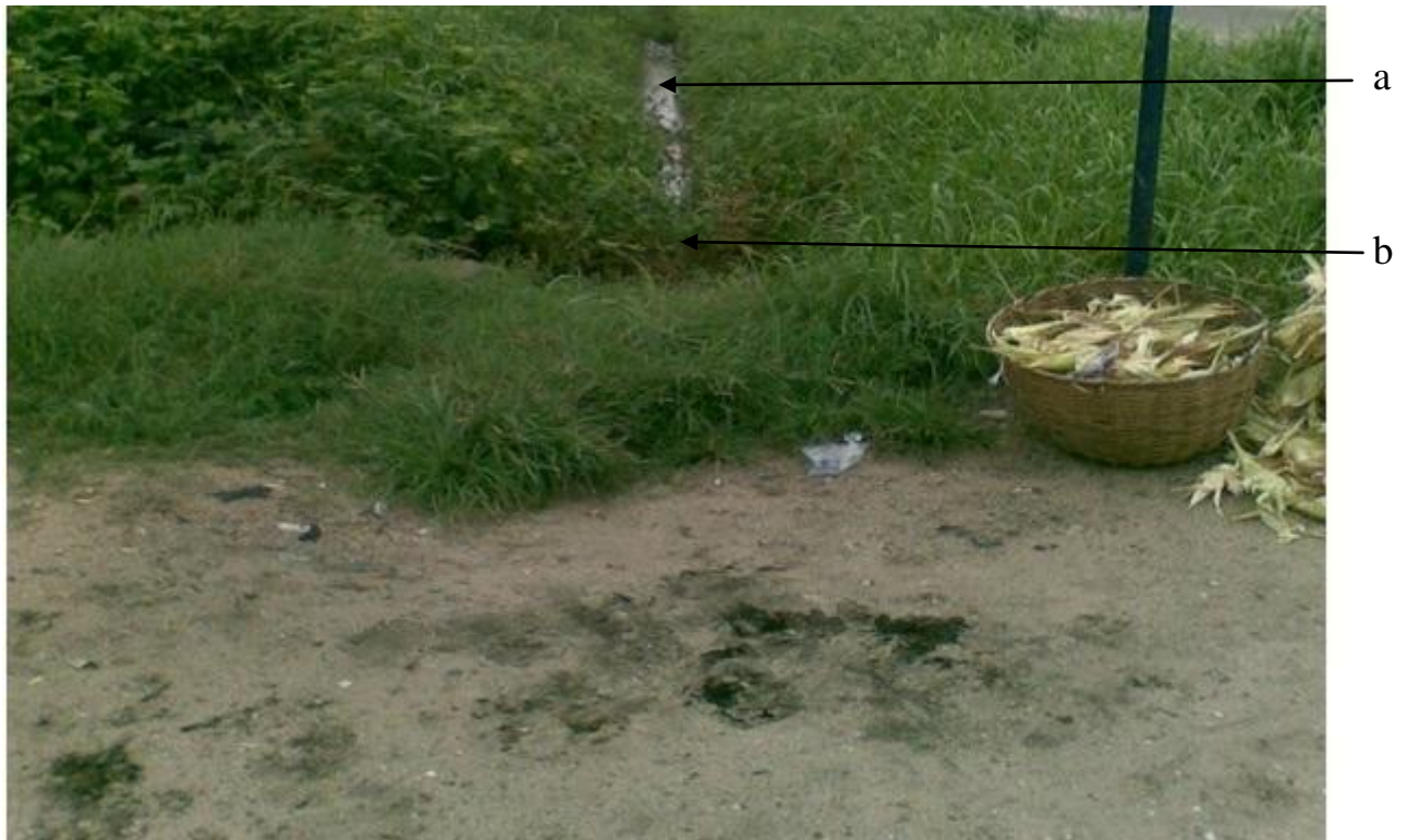
An occluding wastewater drain on Ahmadu Bello Road in June, 2004 with (a) gradual loss of habitat to wastewater fauna including P. reticulata and (b) fully blocked section.
