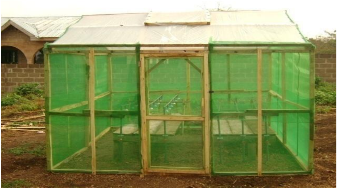
Plate 2: Front View of the greenhouse
