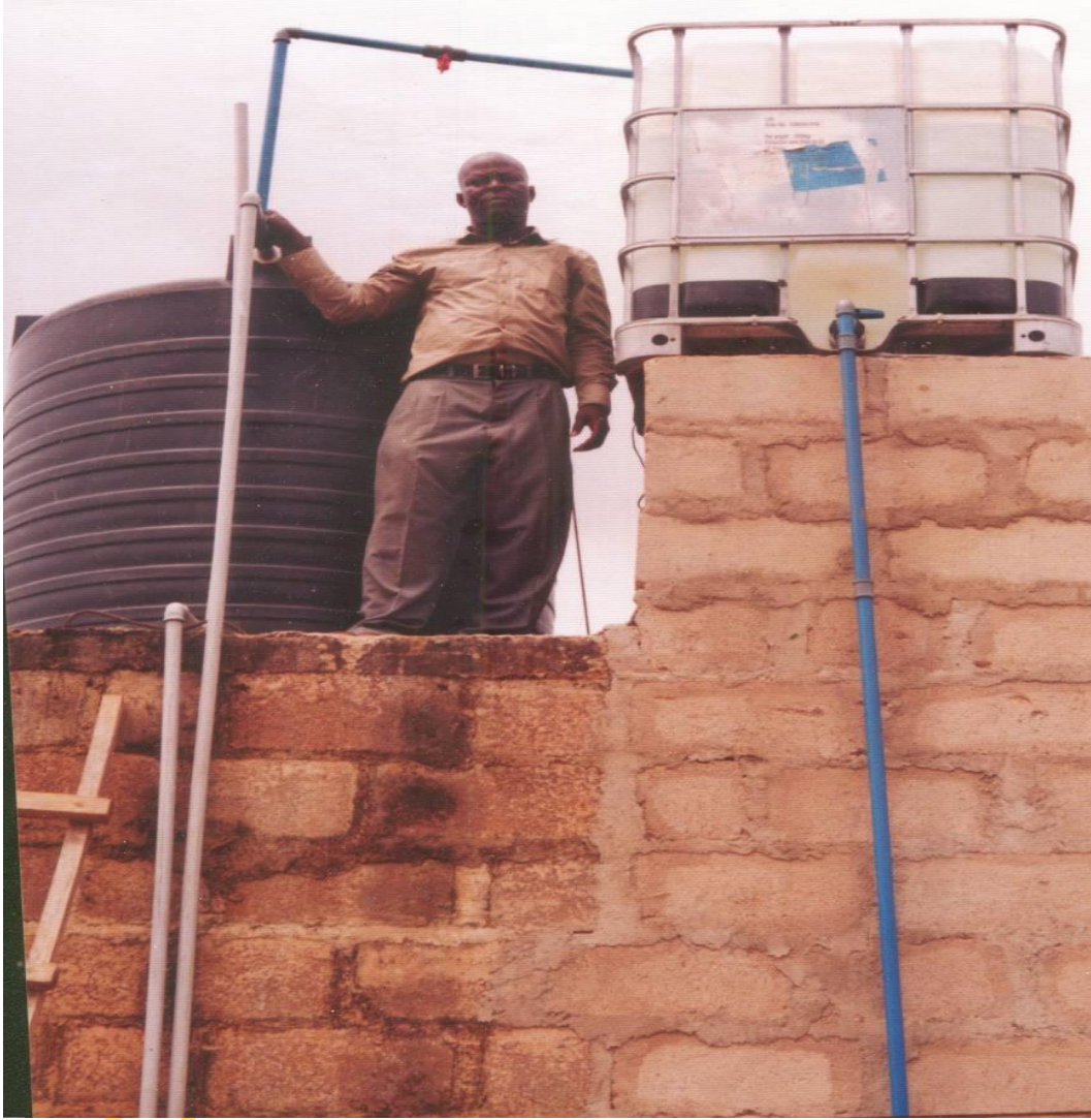
Plate 7: Rubber tank placed on the scaffold
