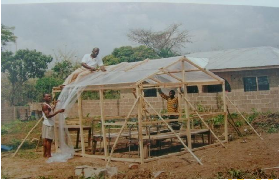
Plate 4: Roof of greenhouse being glazed with polyethylene film
