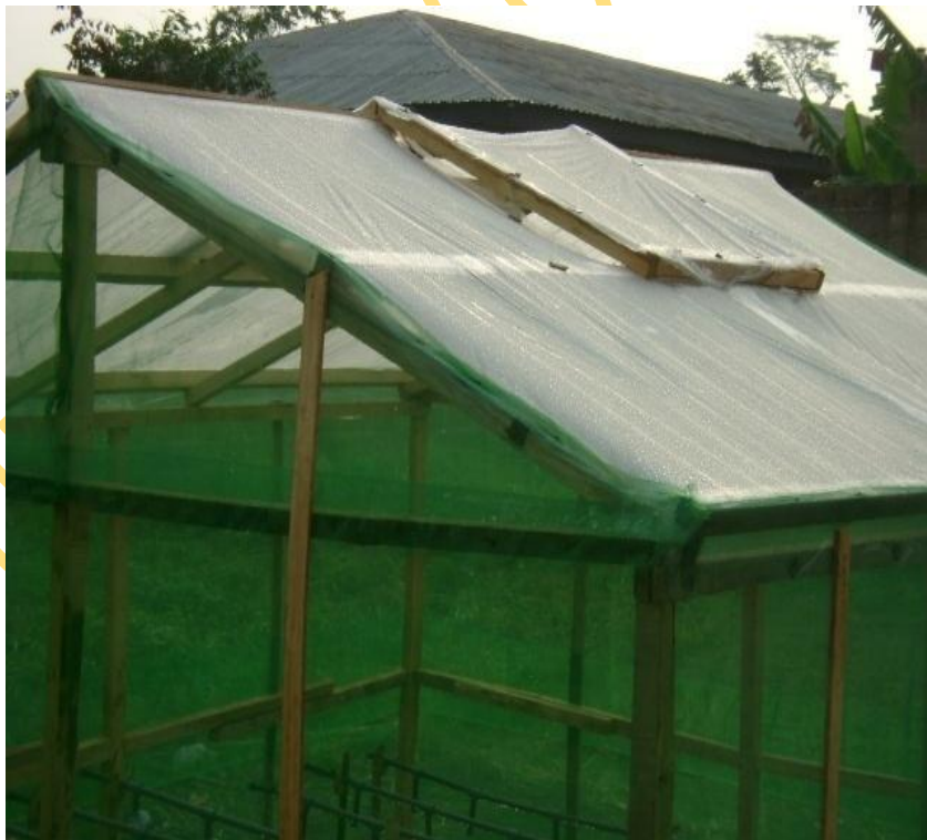
Plate 5: The gable roof with vent
