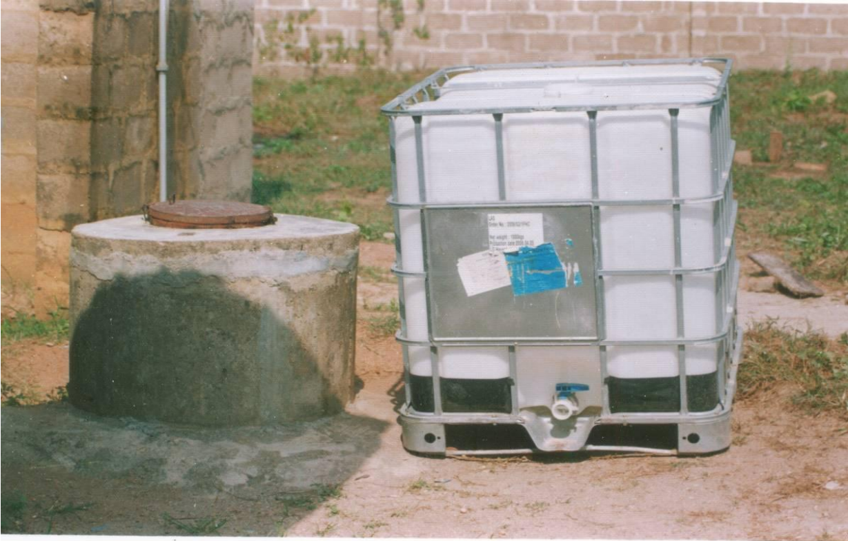
Plate 1: A 15.6m deep well operated by a 1 1/2 horse power DP-151 DAF water pump
