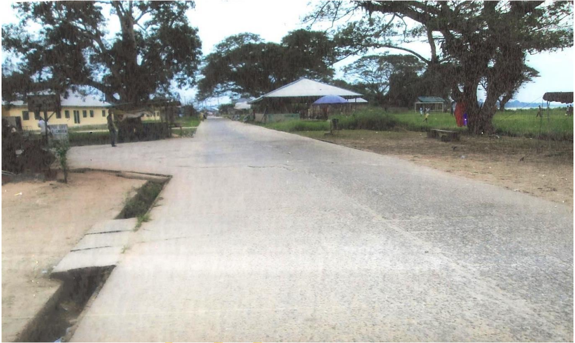
Plate 12. Internal Concrete Link Road, Odi
