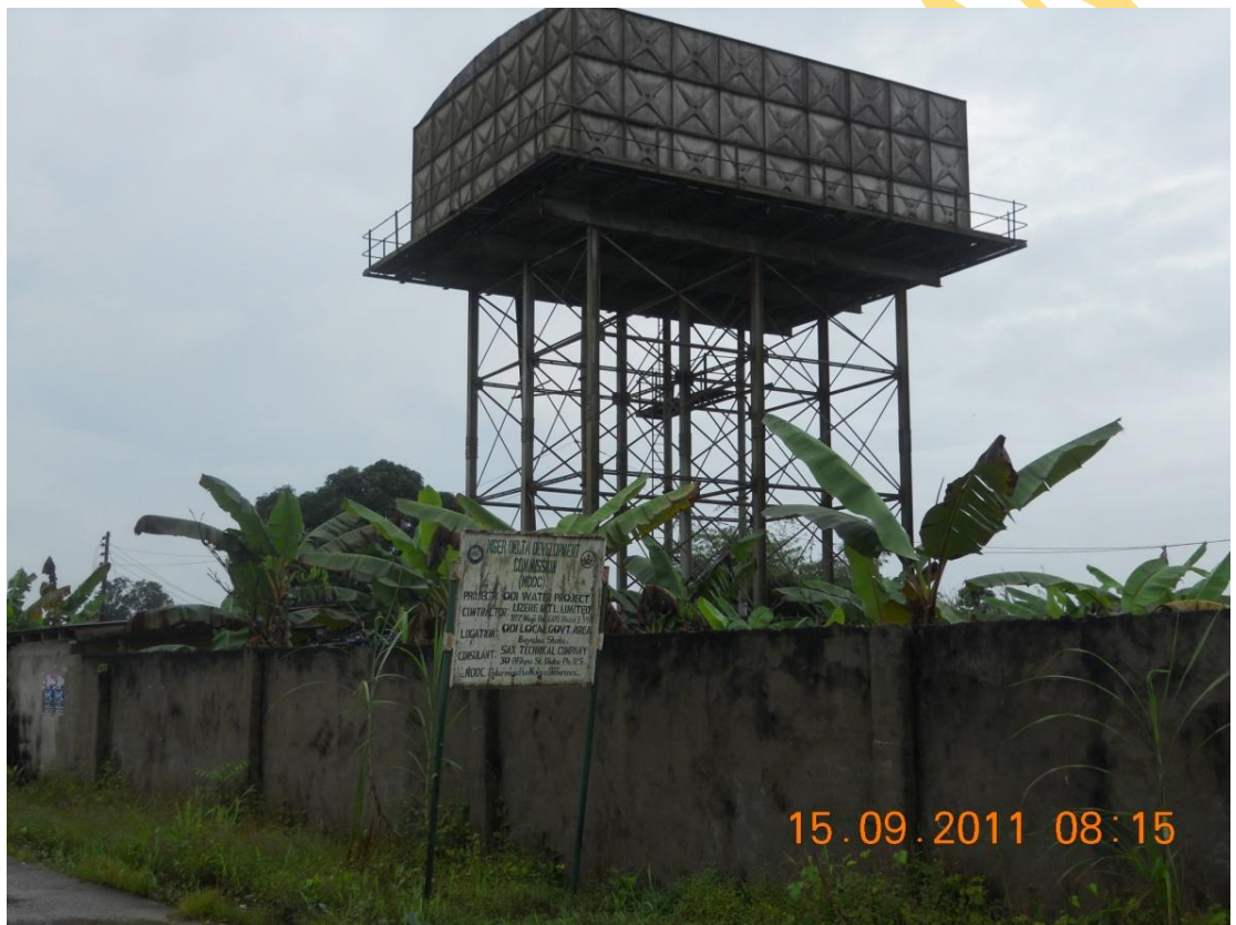
Plate 9. NDDC Water Project in Odi
