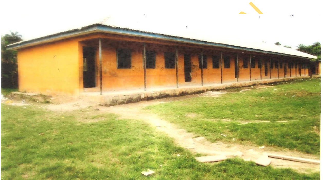
Plate 13. A Block of Six Classrooms at Government Secondary School, Odi
