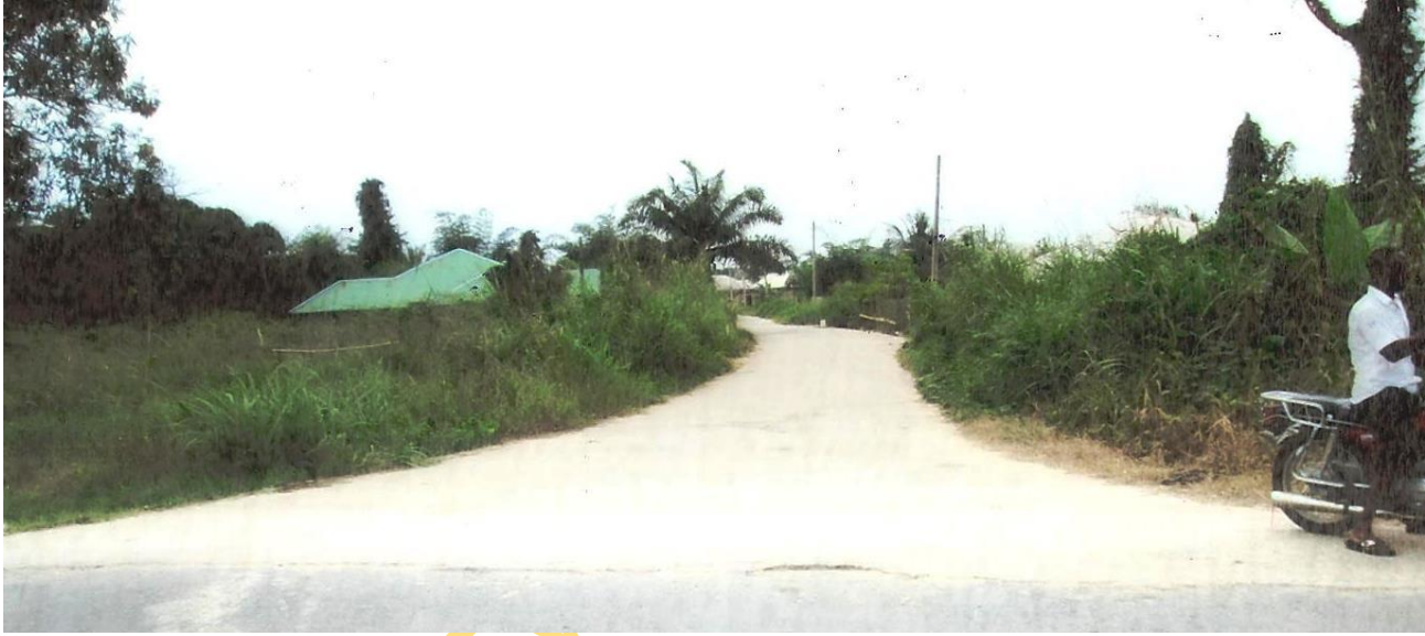
Plate 11. Odi Internal Concrete Link Road by the Women's Leader's House
