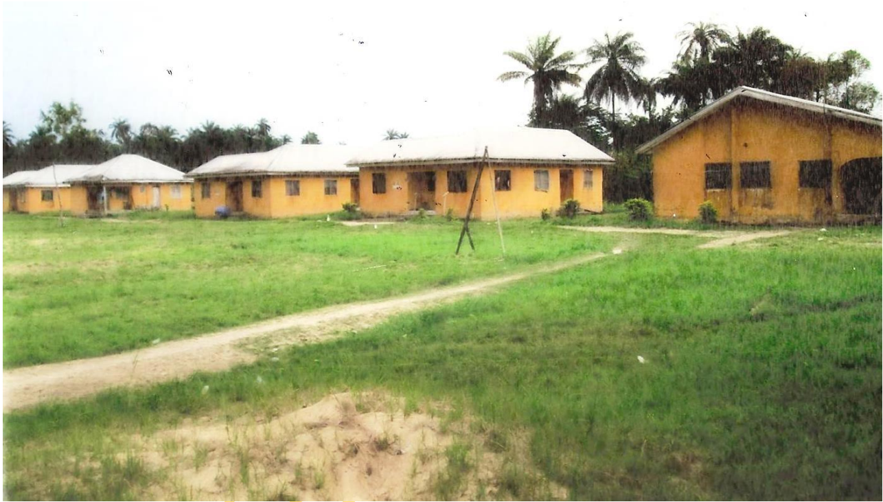
Plate 15. Staff Quarters at the Government Secondary School, Odi
