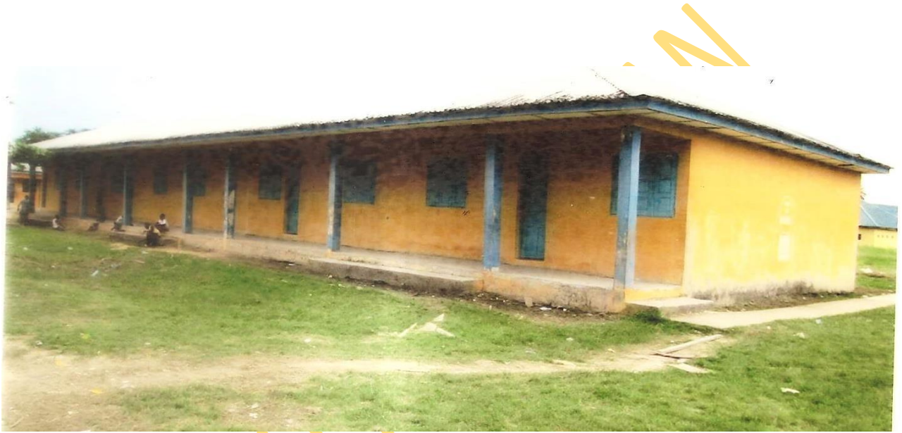
Plate 14. Six-room Science Laboratory at Government Secondary School, Odi
