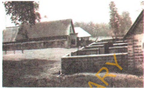
Pig house in a cleared area of the farm
