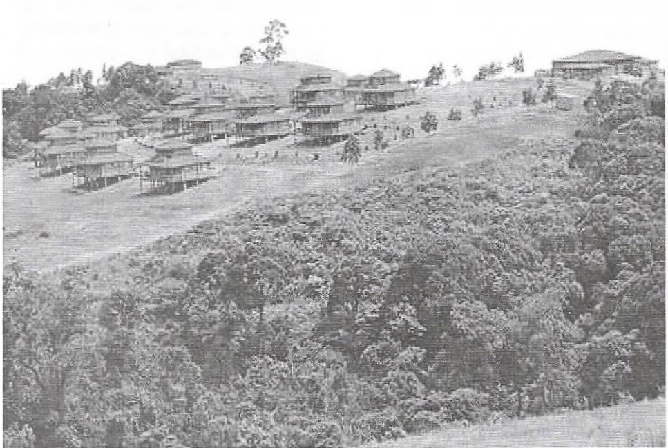
Plate 1: Mountain Villas at Obudu Mountain Resort
