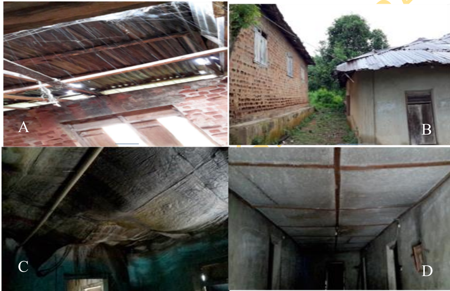
Figure 3.3: Common houses and ceilings at Akaka-Remo. a) Mud and un-cemented houses with no ceiling. b) mud and cement houses are always in sympatry at Akaka-Remo. c) another common ceiling at Akaka-Remo (mostly detached). d) few houses have ceiling and cemented walls at Akaka-Remo
