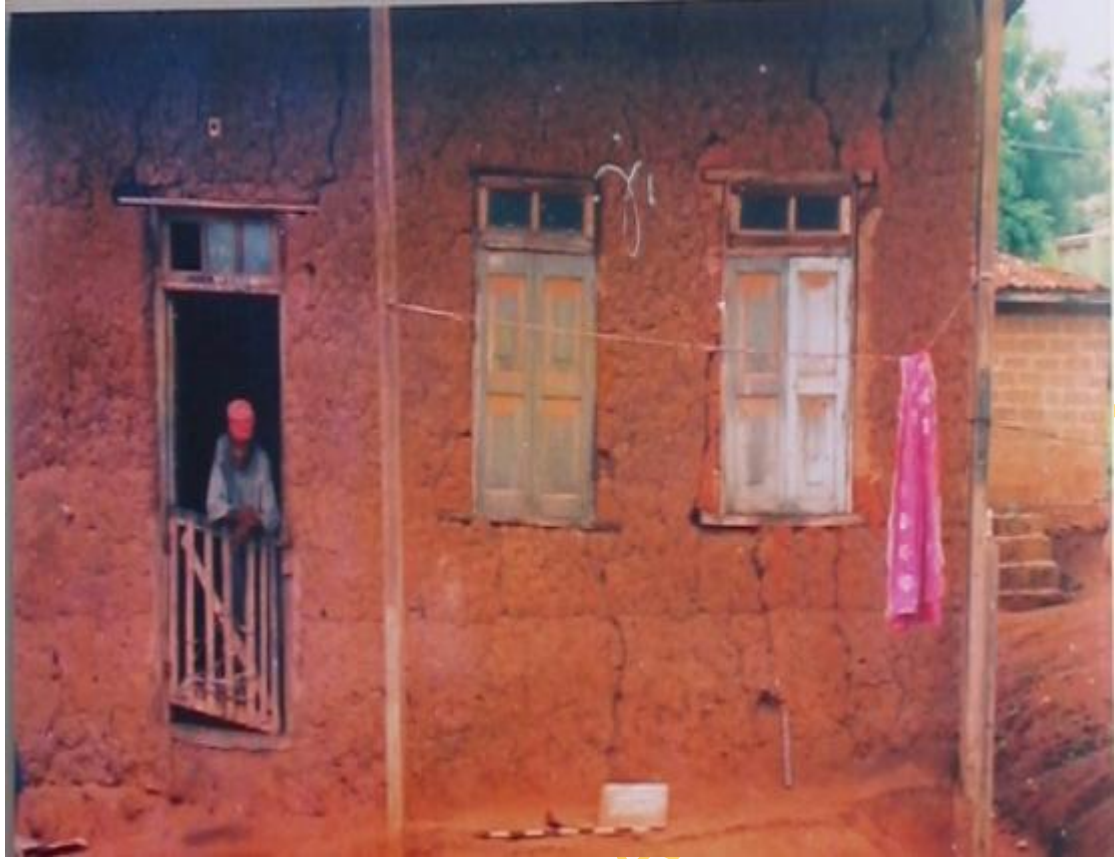
Plate 3.12: A building over the Iragbiji pavement
