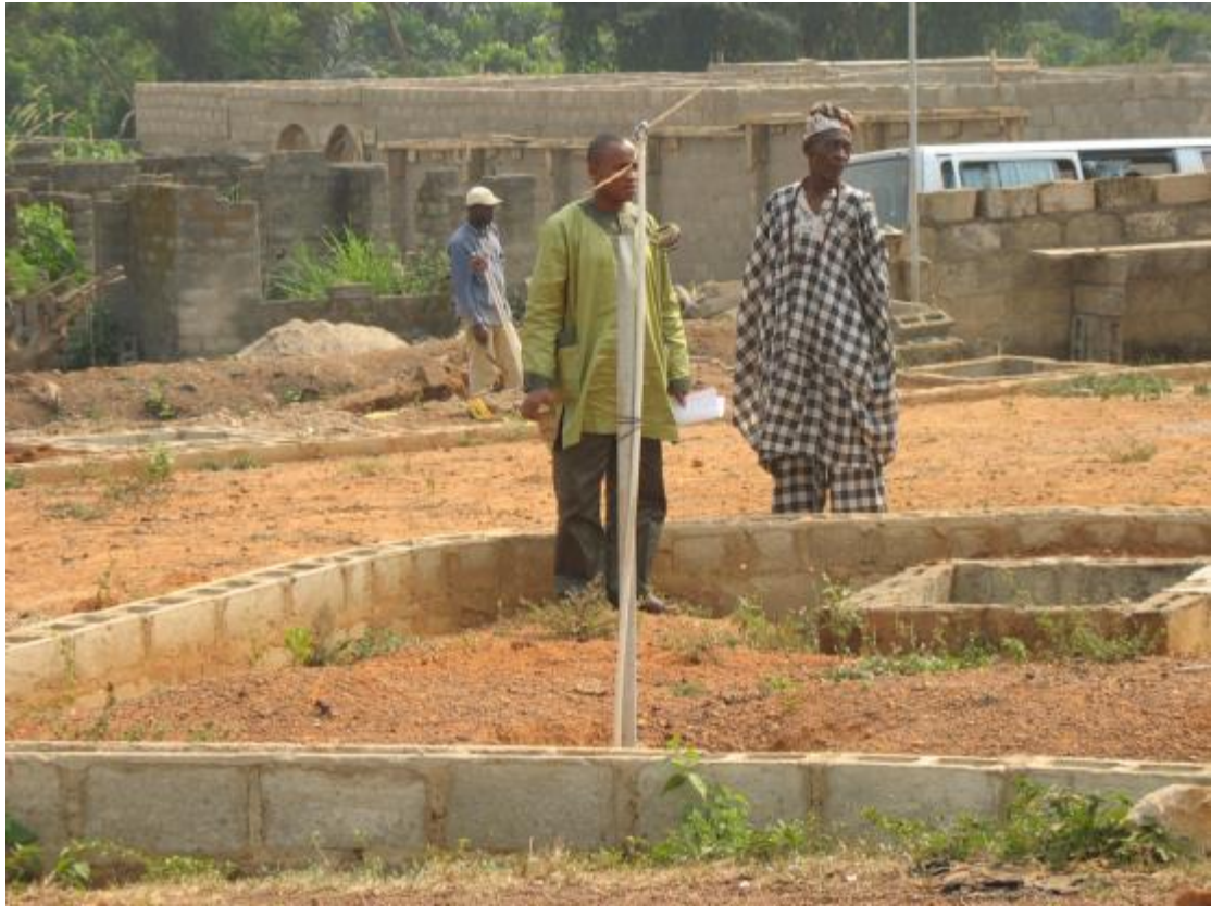
Plate 4.2: Petrol Station under construction on the Ila-Orangun potsherd pavement site
