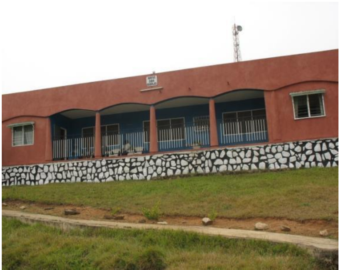
Plate 3.4: Igbajo New palace building
