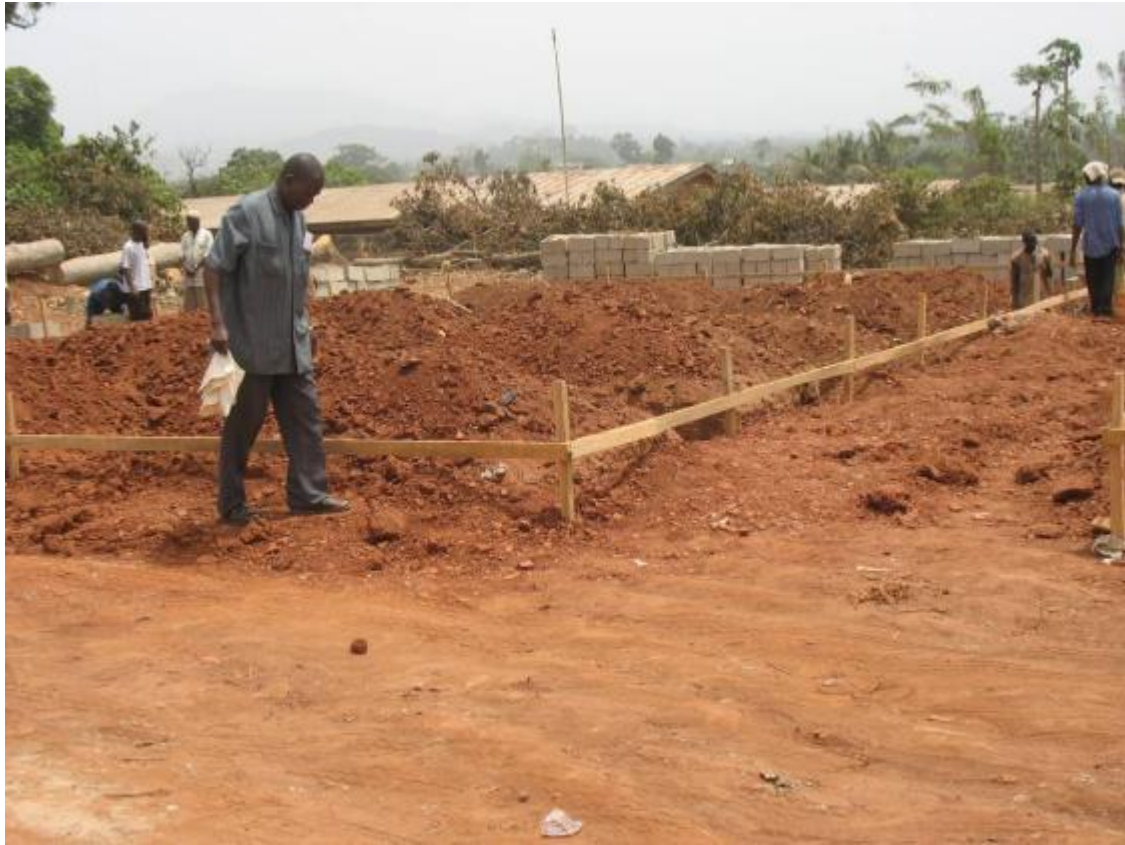
Plate 5.25: A building under construction at Ita-Yemoo, Ile-Ife
